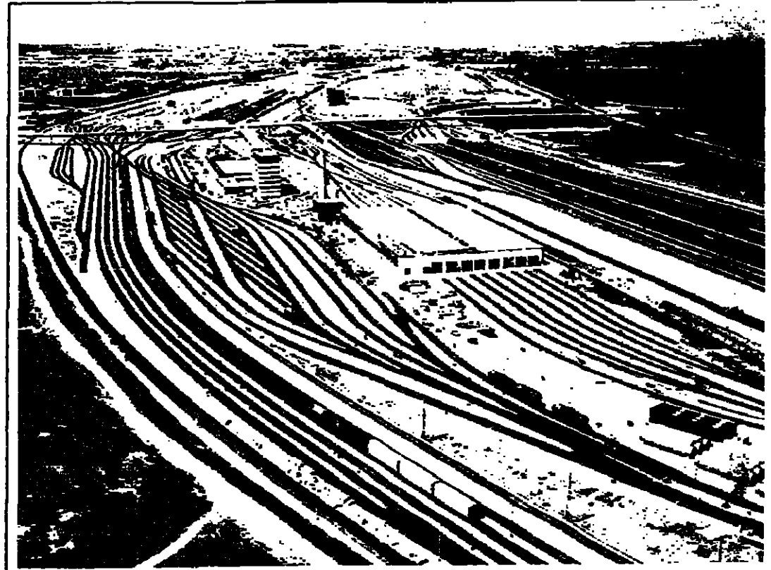
HAMBURG INAUGURATES EUROPE'S LARGEST RAIL JUNCTION -- This bird's-eye view of seven years' hard work, inaugurated on 7.7.77, conveys some idea of what will soon be Europe's largest and most up-to-date railway shunting yards at Maschen, near Hamburg, Germany. The complex is seven kms. long, 700 metres wide and has cost 770 million Deutschmarks. Ninety-five per cent of rail freight converging on Hamburg from Scandinavia, overseas and the north of Geneva, will in future reach its destination within 36 hours. Goods bound for Munich or Basle, for instance, will reach the customer a full 24 hours earlier than at present.
